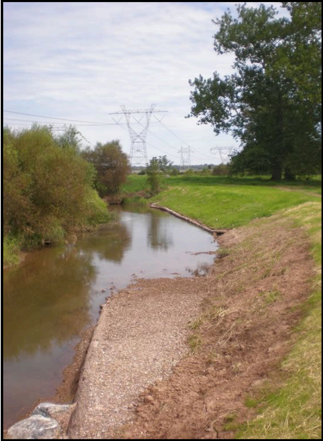
Photo 1. 2009 “Before” photo of Conewago Creek at Hershey Meadows site, shortly after implementation of a log vein deflector and a mud sill. Photo Credit: Jim Shortle
