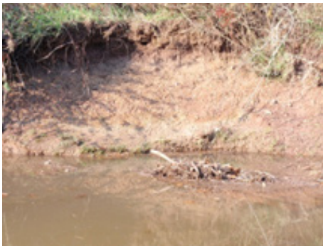
There is no vegetation on the bank. Banks may be steep with evidence of severe erosion.
